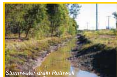
Stormwater drain Rothwell
